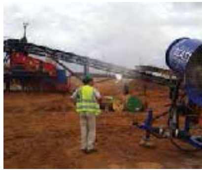
2 Dust suppression at RHC
