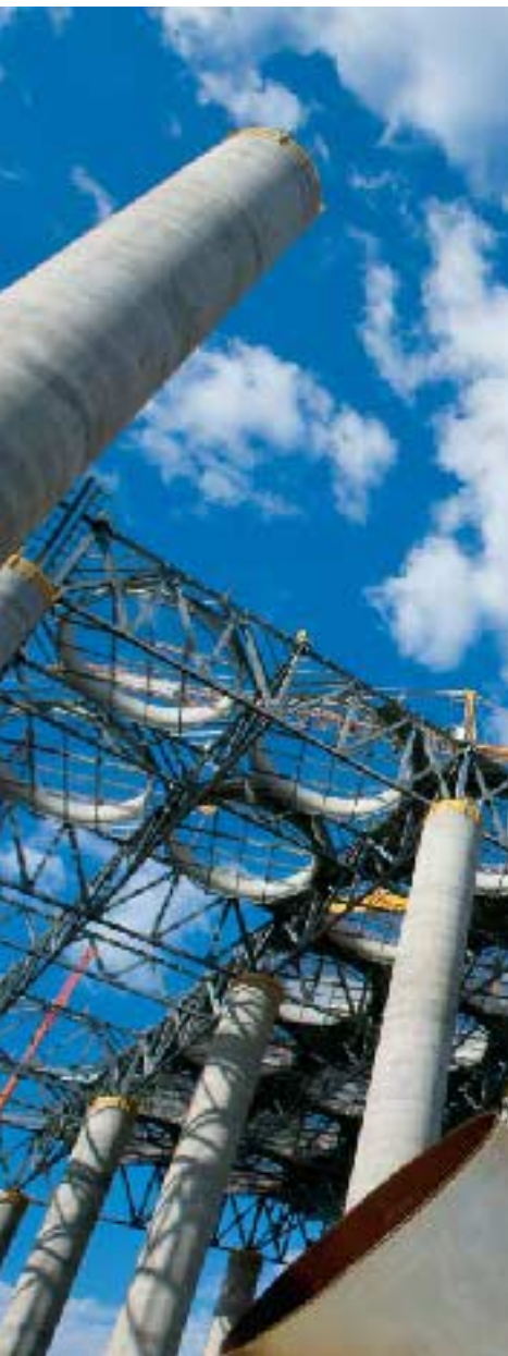
Medupi power station air cooled condensers
