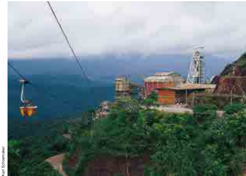
This headgear belongs to Cuiabá, one of the mines in Brazil which AngloGold acquired from Minorco at the end of 1998. The aerial ropeway is used to transport ore to the Queiroz gold plant, 15 kilometres away.
