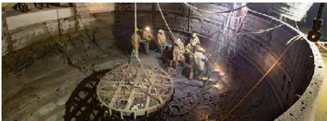
Styldrift Settler No 2 collar construction
