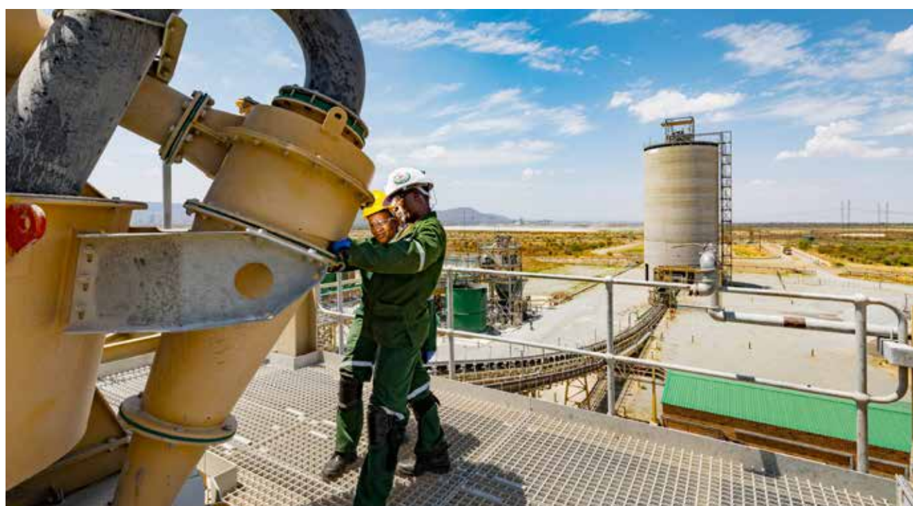
The Cyclone at the Maseve concentrator
