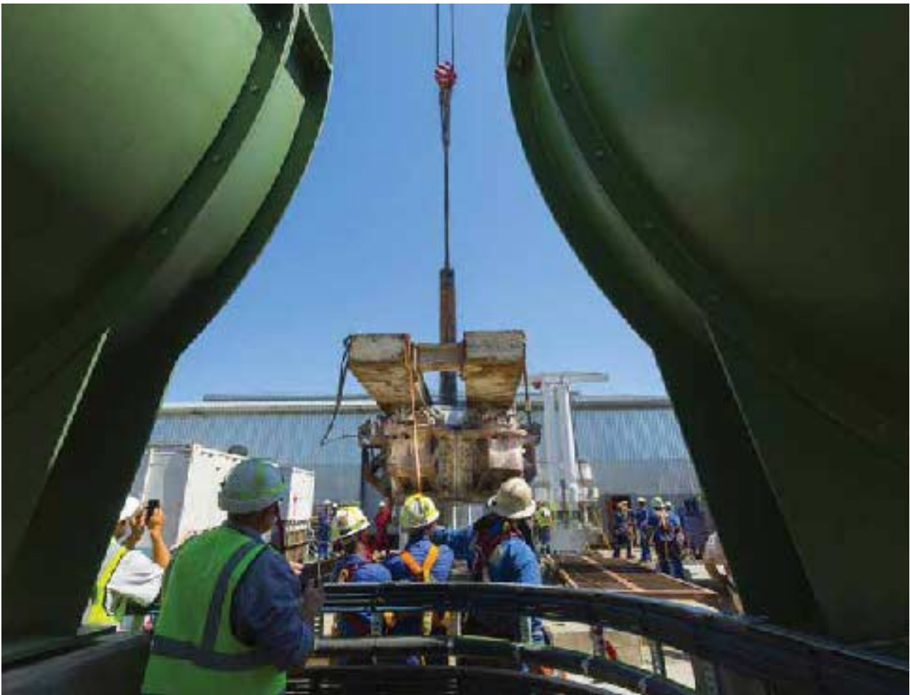
Removal of raise bore machine base after completing reaming of Ventilation shaft I
