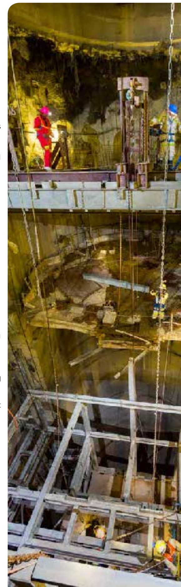
Styl drift I Main shaft loading box construction
