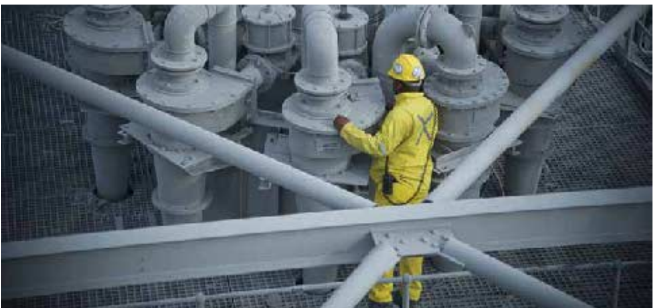
Safety representative inspecting secondary mill cyclone cluster
