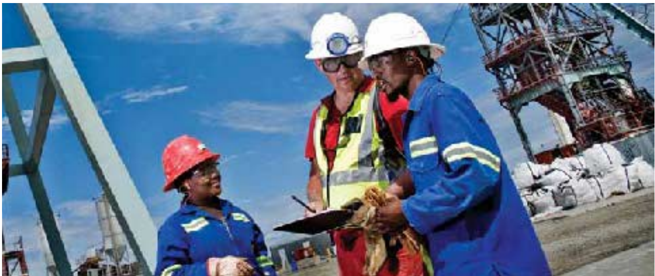
Styldrift I Project under construction
