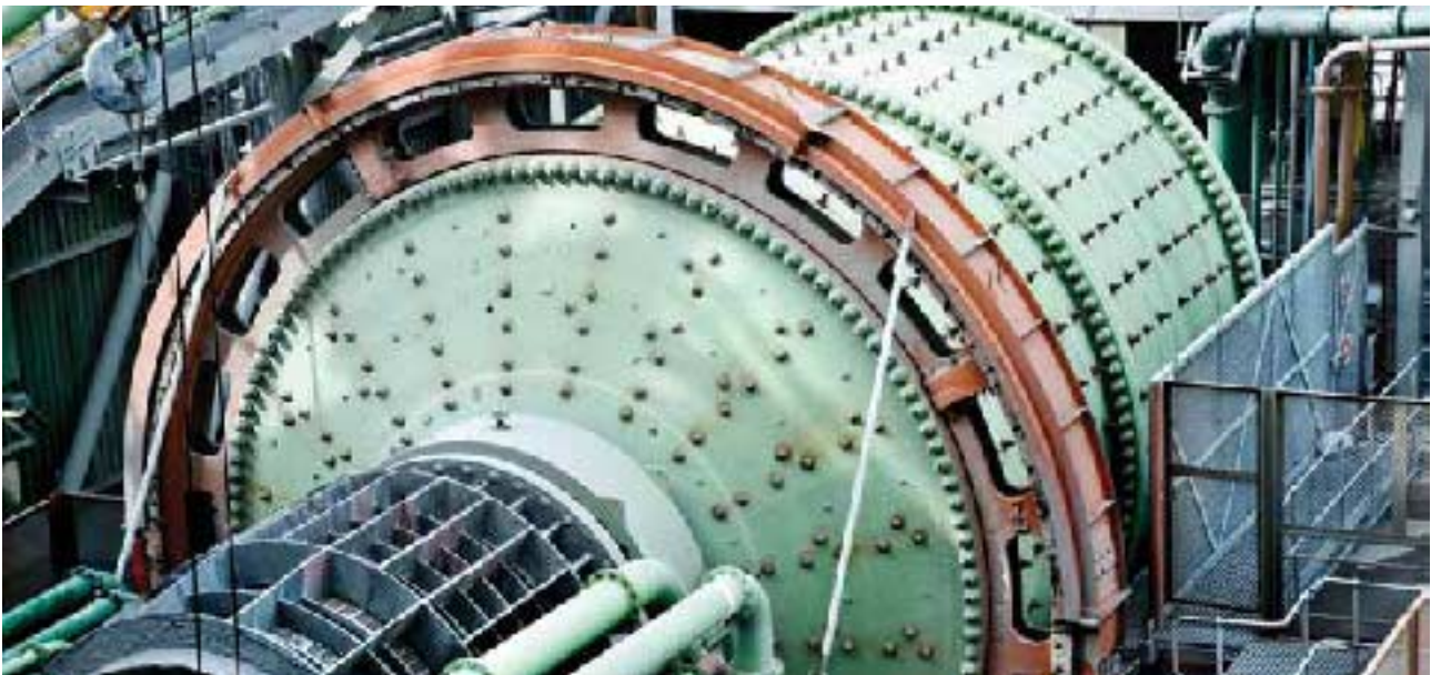
Primary ball mill undergoing routine maintenance
