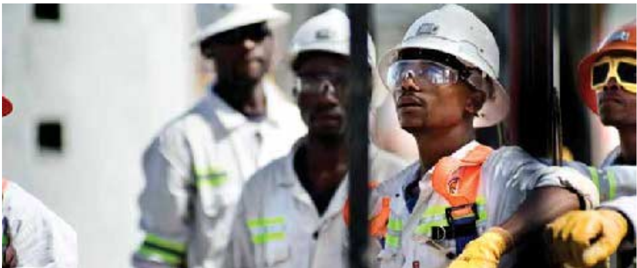
Shaft sinking crew on Styldrift I Project
