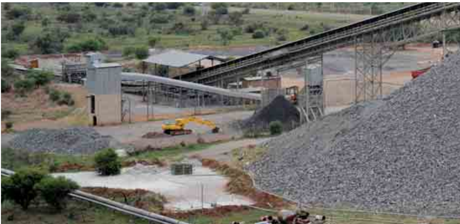
The stockpile offers surge capacity between the mining and plant process
