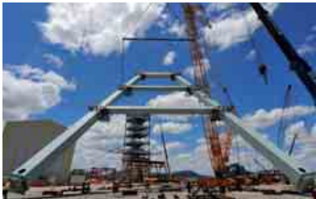
The shaft being sunk at Styldrift I
