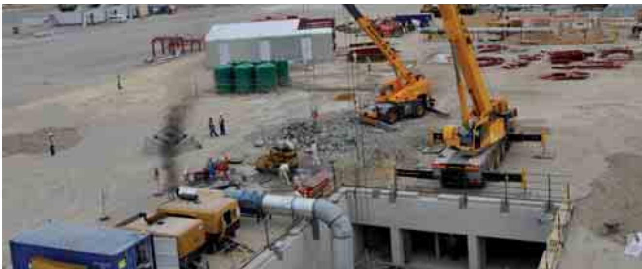
Work underway on the major civil works at the Styldrift project
