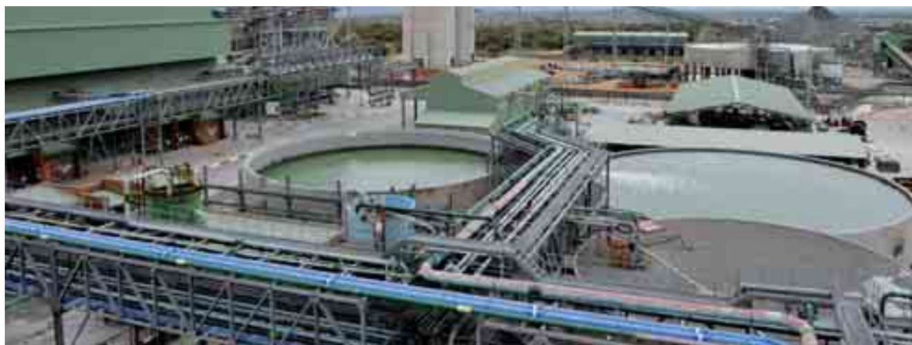
View of BRPM Concentrator Plant
