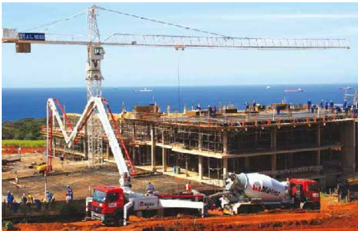
Métier supplying concrete at a construction site in Durban
