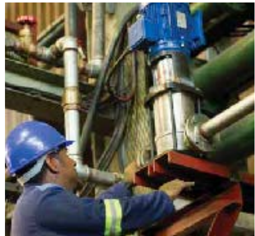
Rowan Moses involved in installing booster pump
