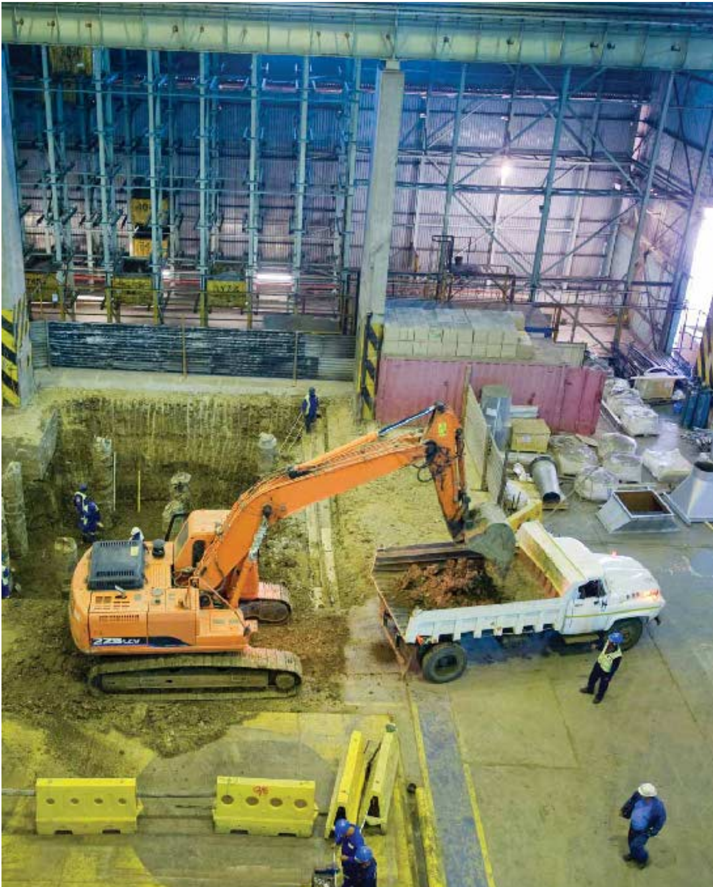
Civils construction for a new charge bucket to be used at the new melting furnace
