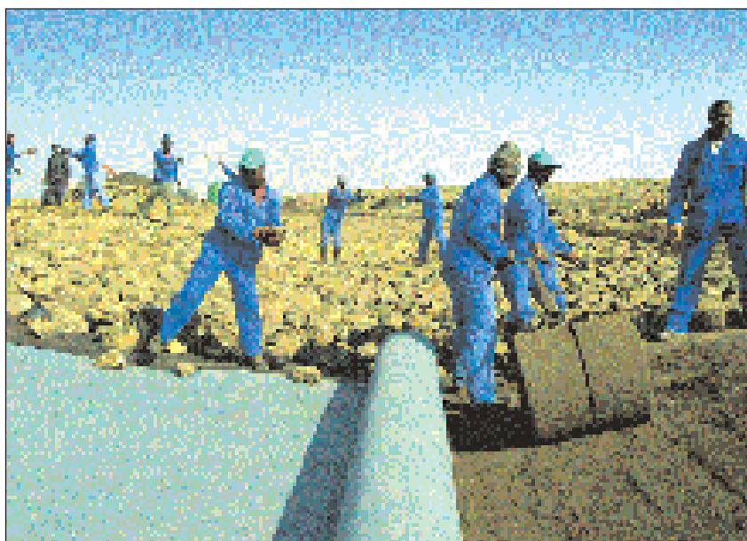
A team sealing the cracks on Hlobane mountain as part of Kumba's pioneering rehabilitation work near the now-closed Hlobane colliery.
