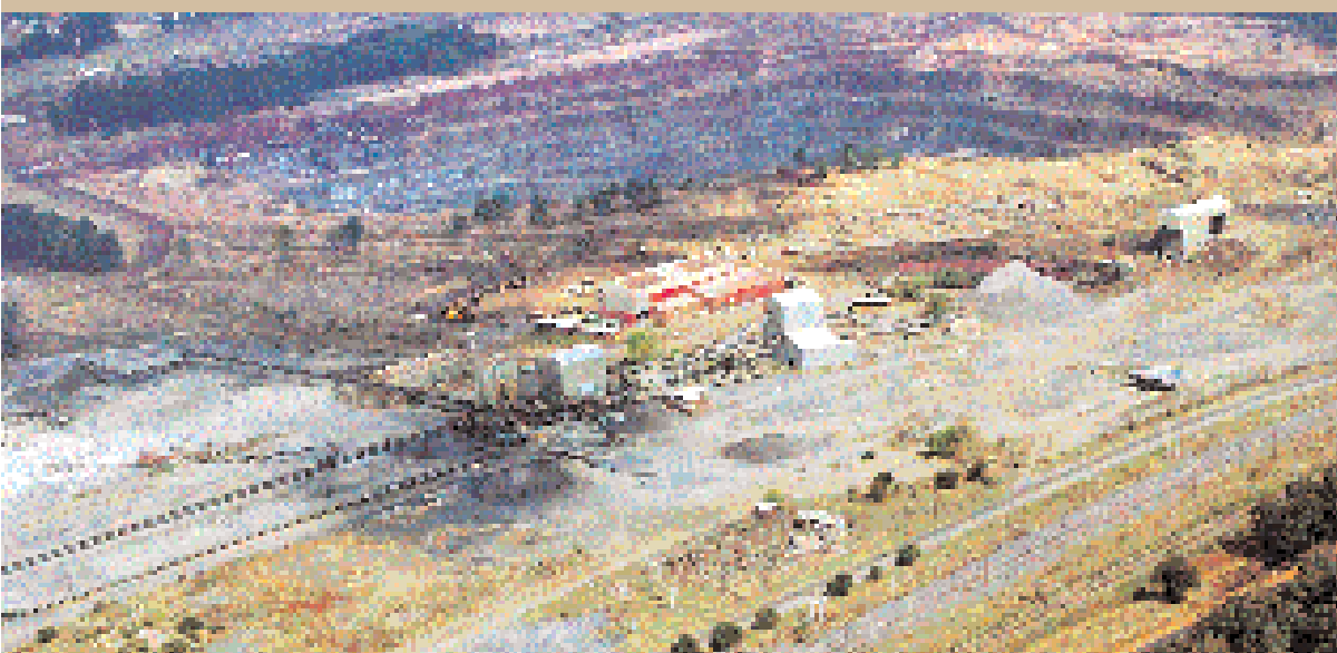
GLEN DOUGLAS MINE
