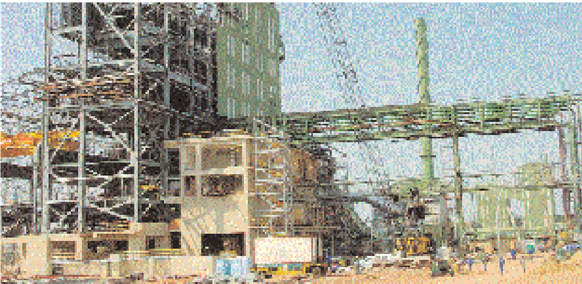
HEAVY MINERALS SMELTER – UNDER CONSTRUCTION
