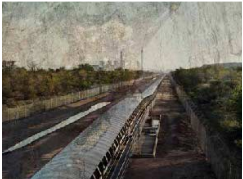
Conveyor belts carry coal from Grootegeluk to Matimba and Medupi power stations. Conveyor belts between the mine and power stations are 4km and 9km respectively
