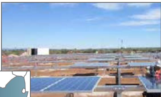
Aveng E+PC – Photovoltaic single-axis tracker for Sishen solar farm, South Africa
