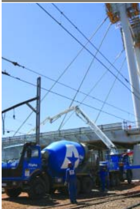
Alpha readymix cement pouring at the Nelson Mandela Bridge
