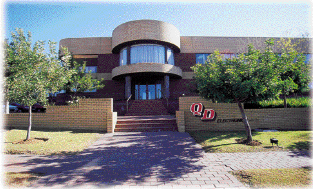
QD House, 91 - 94 Silverstone Crescent, Business Park, Kyalami
