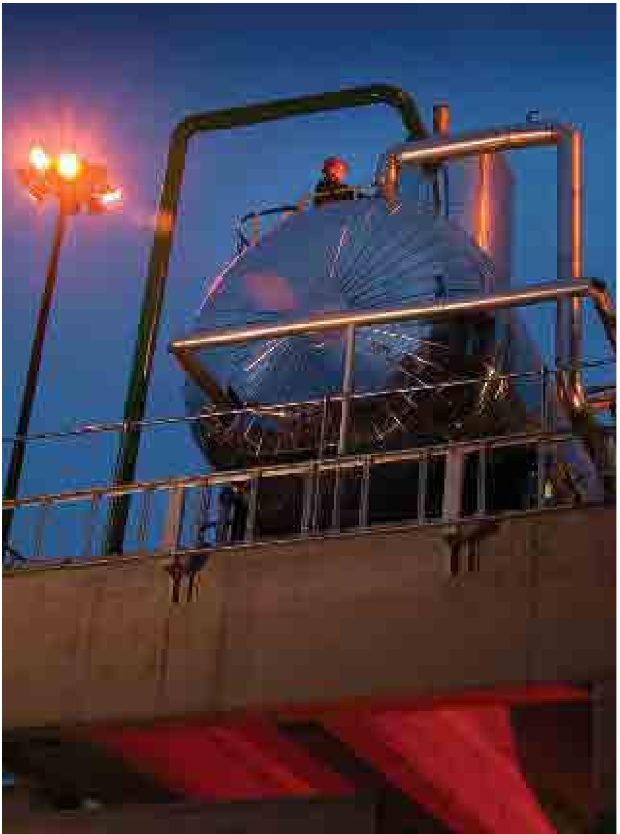
Alwyn Botha checking pressures on the newly commissioned deaerator section of the ancillary equipment for boiler 7 at RBMR.
