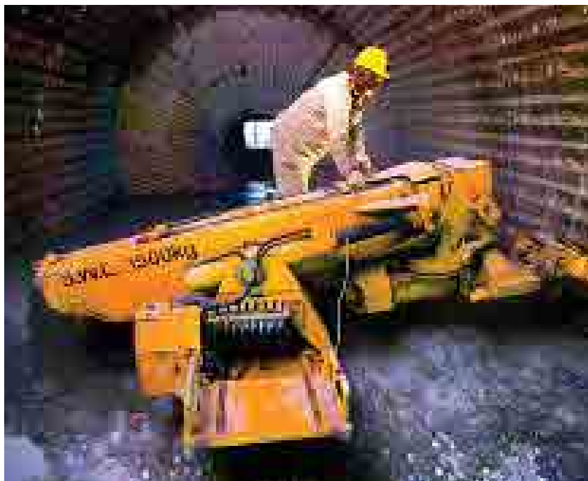
Joseph Lesetja Rafam conducting maintenance on the interior lining of the ball mill at the PPRust concentrator.
