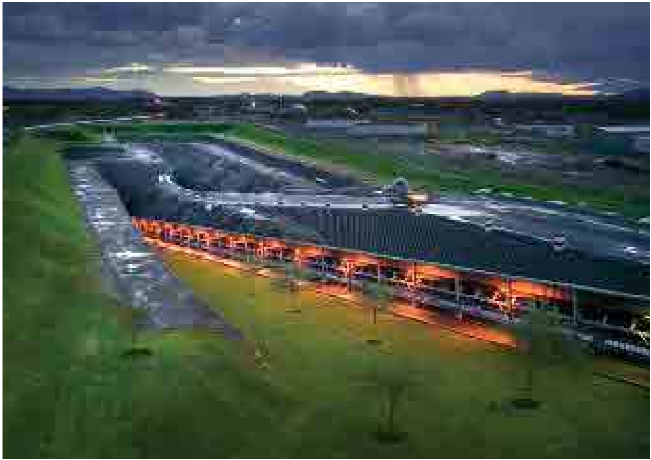
The 4B Shaft portal at Union Section.
