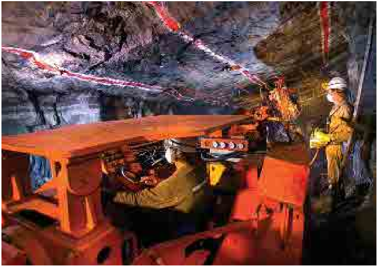
Roof bolting via remote control in progress.
