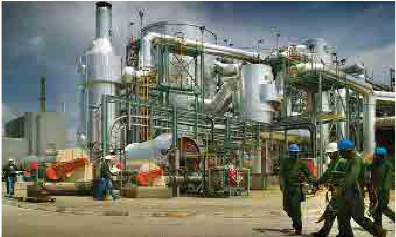
The new double-contact double-absorption acid plant at Waterval Smelter that will allow 99% fixation of sulphur and SO 2 emissions to drop below 20t/day.
