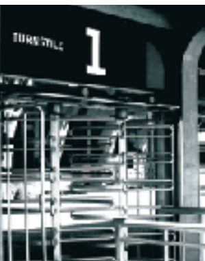
Johannesburg Soccer City stadium stainless steel turnstiles
