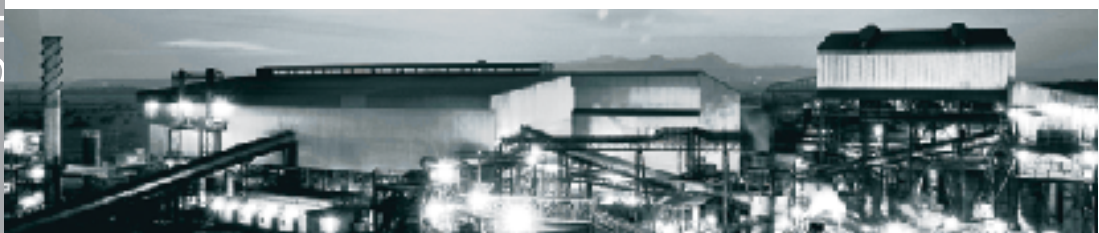
The Bokamoso pelletising and sintering plant, North West province
