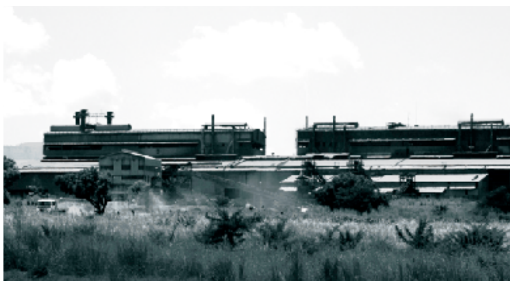
Wonderkop ferrochrome plant, North West province
