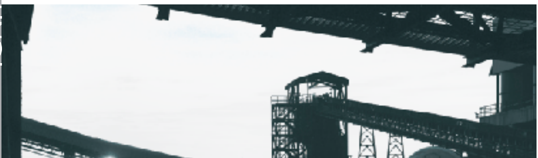
Bokamoso pelletising and sintering plant in the North West province
