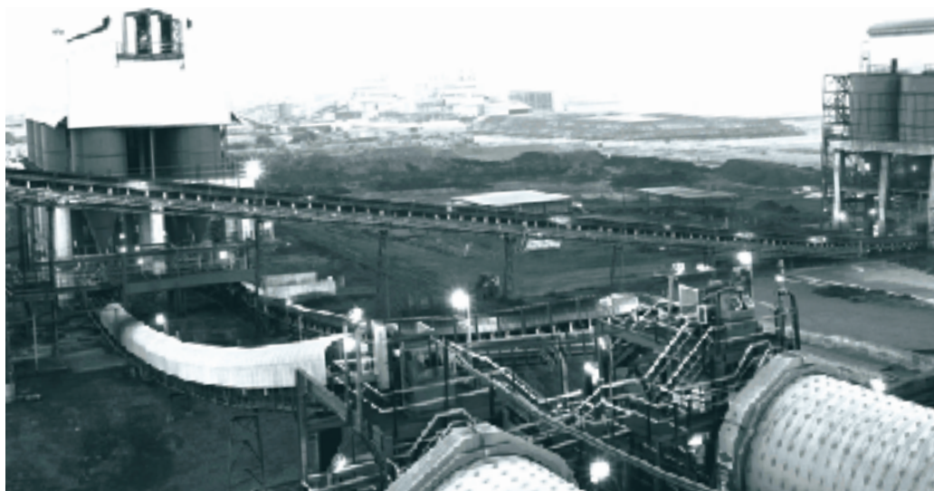
Bokamoso pelletising and sintering plant, North West province
