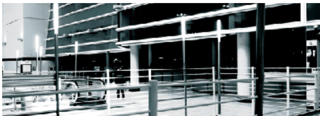
Another example of the use of stainless steel in a Gautrain station
