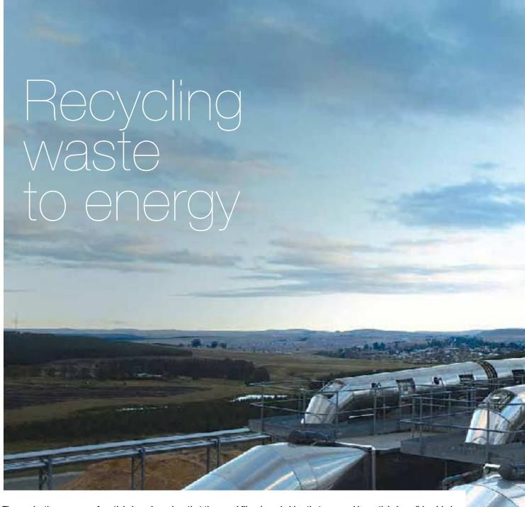
The production process of particle board requires that the wood fibre (wood chips that are used in particle board) be dried before it enters the production process. The resin that is used to bind the particle board also needs to be heat activated after the particle board mattress has been compressed. To supply the heat needed for these two processes, a 45 Mw step grade thermal energy plant was specifically designed and built for PG Bison's production facility in Ugie.
