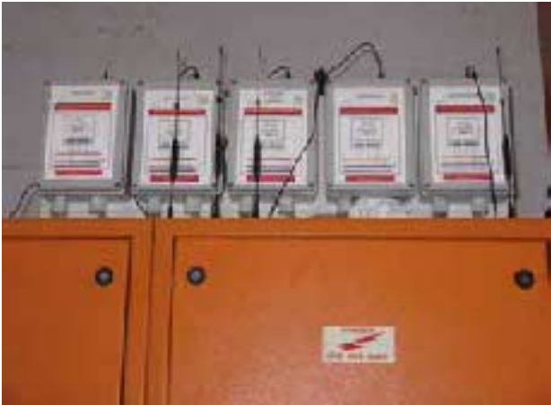
Installation of Powerstar electricity meters which record consumption per second: this allows us to increase production during low peak periods
