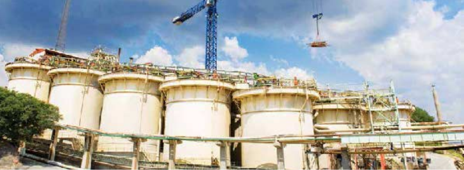
Above: CIL circuit at Ergo's Brakpan plant
