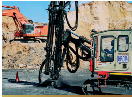
Drilling and Blasting
