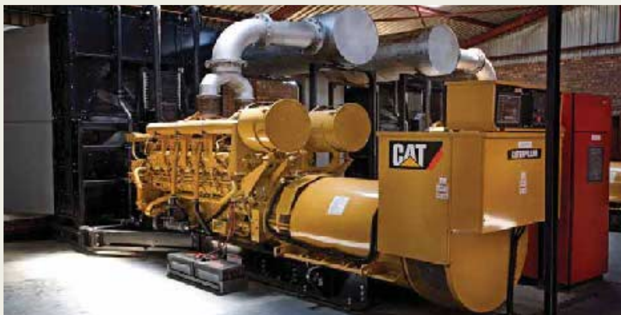
Caterpillar 3516 unit with a 2 500 kVA, supplied and commissioned by Barloworld Power at a coal colliery
