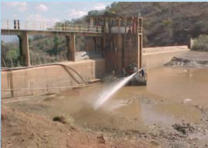
A view of the Mapochs Dam desilting process
