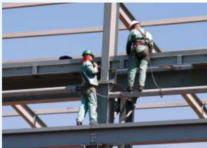
Rapid erection of steel framed building using Highveld beams for the new ferrovanadium plant
