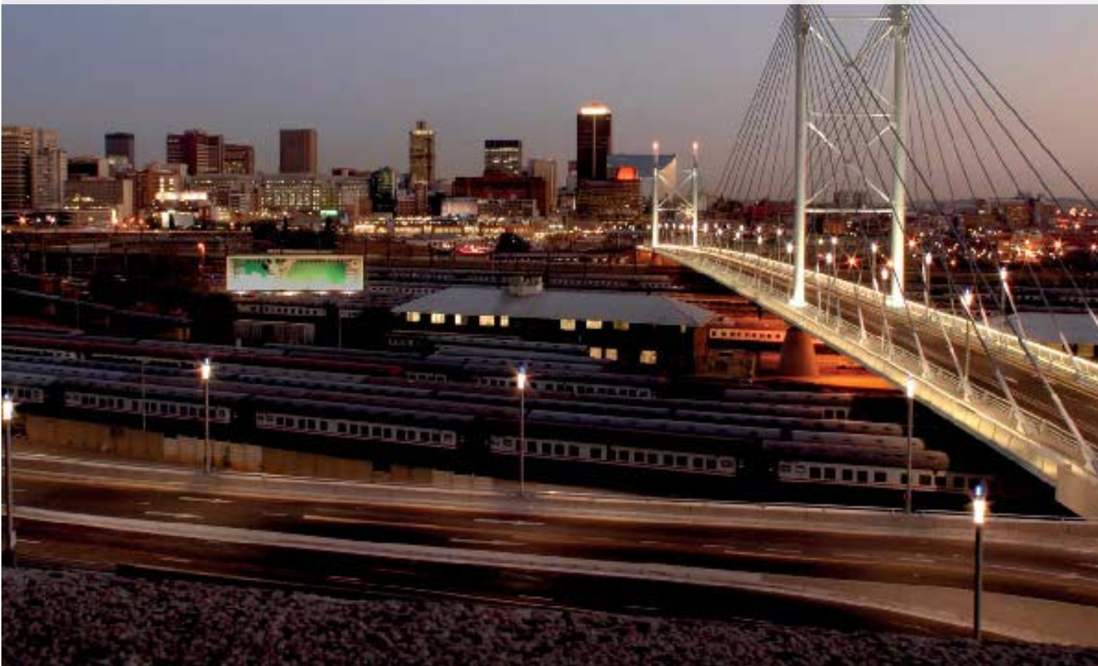
Johannesburg Nelson Mandela bridge
